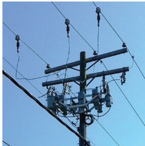
Figure 4: Optisense MV Optical Current & Voltage Sensors attached to 3 Phase Distribution Lines
