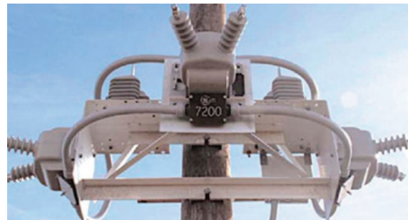
Figure 3: GE Voltage & Current Transformer (PT/CT)
